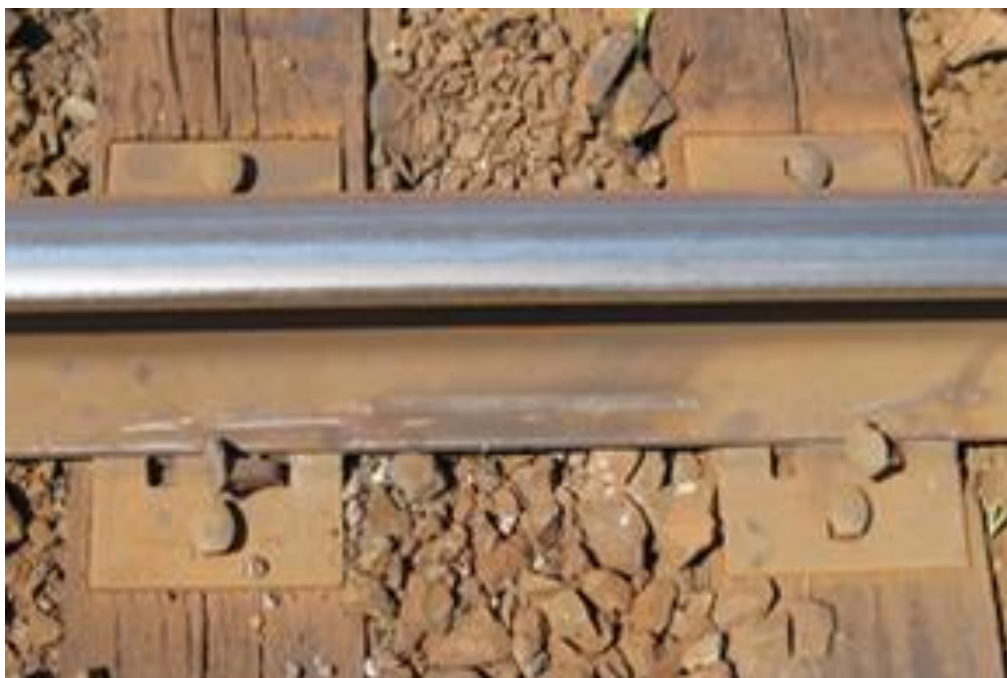
Figure 3-6: Bent and lifted gauge-side low rail spikes at the point of derailment
